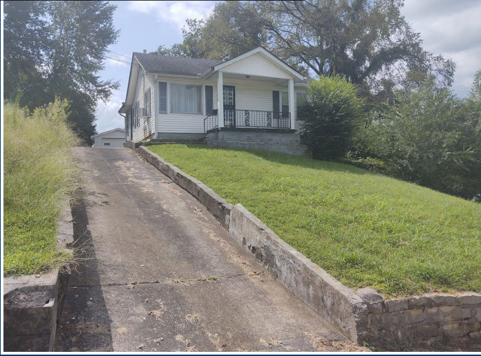
PROPERTY#1 - 212 THIRD AVE E
